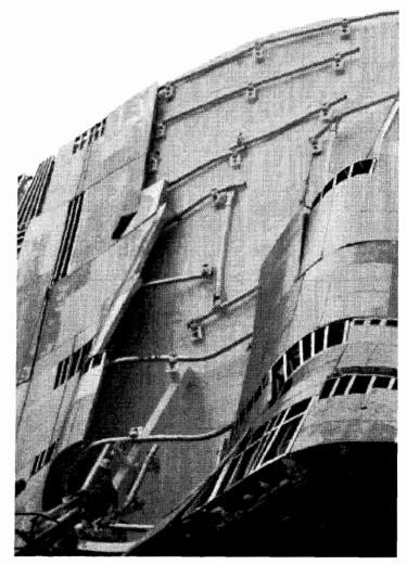
Figure 4. EMP cladding under construction – steel pipe support structure over shot-crete (photo by Eric Olson)
